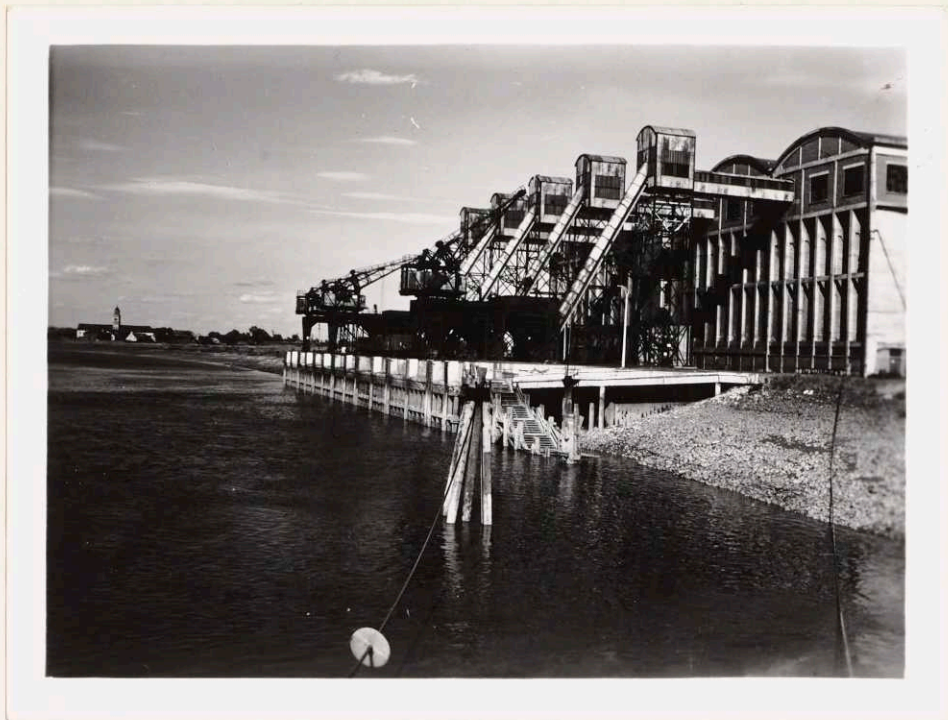
COAL CONVEYORS & BUNKERS @ INTERESCAUT
