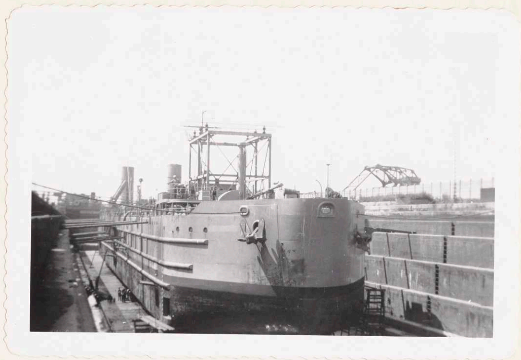
INLET TO RAW WATER SYSTEM
